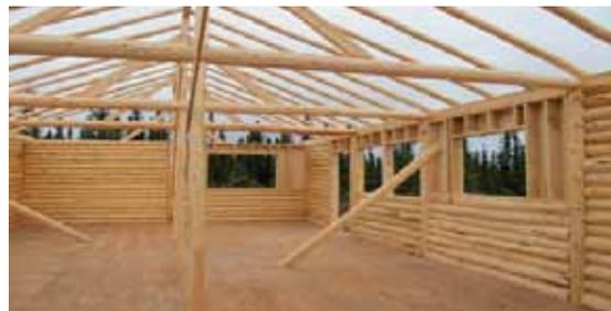
The Log Cabin Building Training Program was a project that required a lot of hard work and long hours. Harvest the logs without the help of machines like ATV or snowmobiles took most of time. The following is the Log Cabin Building process that was followed to construct the 20 x 40 Log Cabin.
